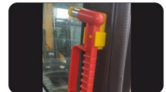
Safety Hammer & Fire Extinguisher
